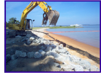
Harrison Road Shoulder Stabilization on the James River– Ft. Eustis
