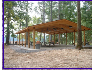
Ft. Eustis Picnic Shelter
