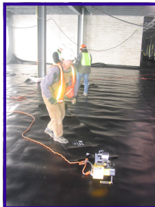
Installation of Vapor Control System Membrane Layer Bayshore Mall, Glendale, WI
