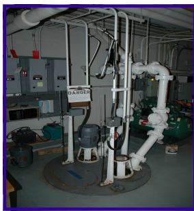
USDA Morgantown Sewage Pump Replacement Morgantown, WV
