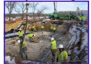
Footing Installation Ft. McCoy, WI
