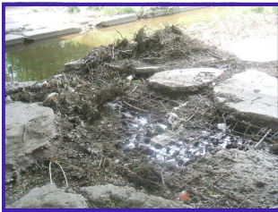
Example of Liner Cracking at Various Channels, Milwaukee, WI
